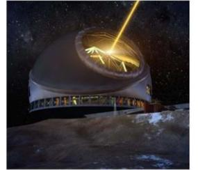
Shows a rendering of the Thirty Meter Telescope during nighttime operations using the Laser Guide Star Facility (LGSF). The LGSF will create an artificial star, with a laser beam directed at the telescope. The LGSF will create an artificial star, with a laser beam directed at the telescope. The LGSF will create an artificial star, with a laser beam directed at the telescope.
